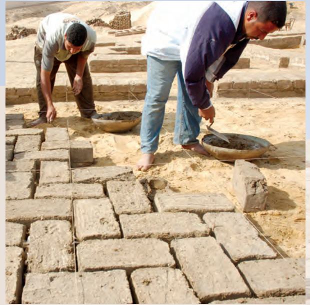
Step 2: We then filled the rooms with sand and laid a mudbrick surface above.
