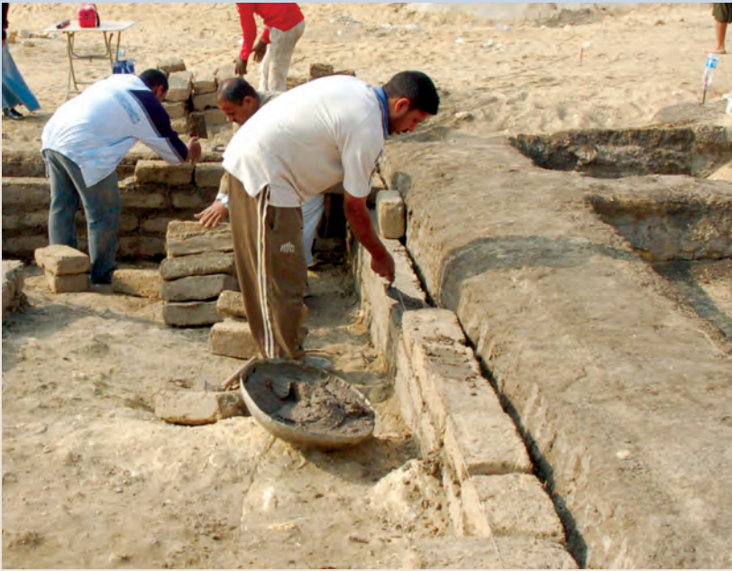
Step 1: We cased the ancient walls with skins one-brick-thick for their protection and to provide the necessary height and stability for the reconstruction.
