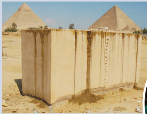
Right: The wall in March 2011, showing damage from ground moisture and rain.
