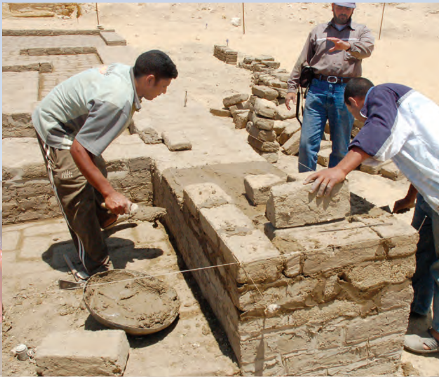
Step 3: We built new internal walls directly above the originals, but with the weight distributed onto the modern skin-walls.
