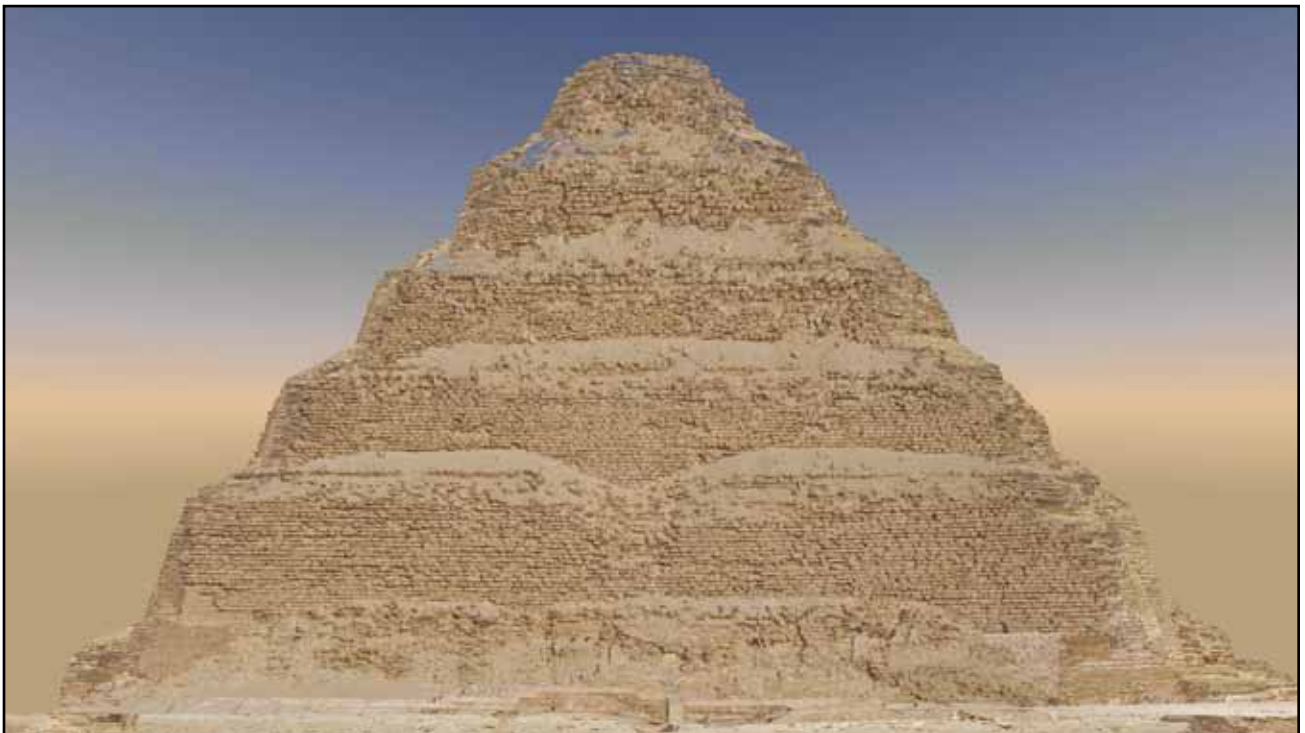
Plate 7.2. Preliminary version of the point cloud model of the Djoser Step Pyramid produced by GLS-1000. Eastern side of the pyramid. Gaps remain until data from the Zoser Scanner are fully incorporated.
