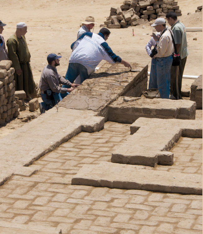
Left: The team discusses how to lay level courses, compensating for the slope by extending successive brick courses northwards as they build up. Note the steep slope of the floor from north (foreground) to south. The floor is covered with brick to protect the original surface and will later be finished with plaster. View to the south. Right: Günter Heindl in the small zigzag rooms that provided a secluded entrance to House E. View to the southeast. Photos by Mark Lehner.
