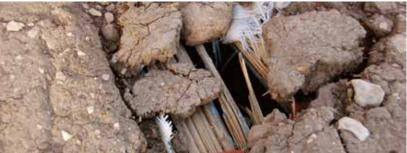
Above: Looking down at a deteriorating roof top in Old Gurna village in Luxor. Mud lies over plant stems. A modern material, plastic, was also incorporated in the roof. Photo by Manami Yahata.
